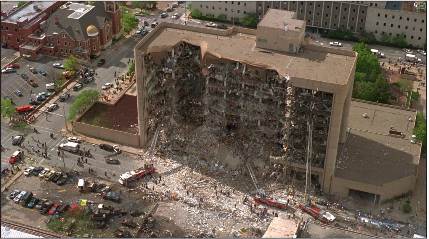
The bombing of the Alfred P. Murrah Federal Building in Oklahoma City on April 19, 1995 was the deadliest act of homegrown terrorism in U.S. history, resulting in the deaths of 168 people. In a matter of seconds, the blast destroyed most of the nine-story building, incinerated nearby vehicles, and damaged or destroyed more than 300 other buildings / Source: FBI
